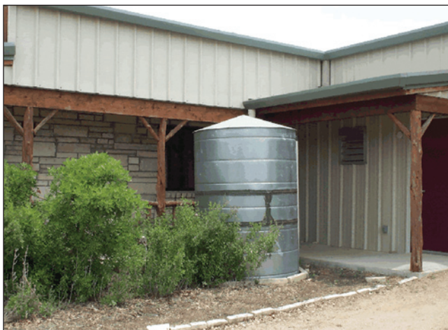
A 2,500 gallon collection tank.
