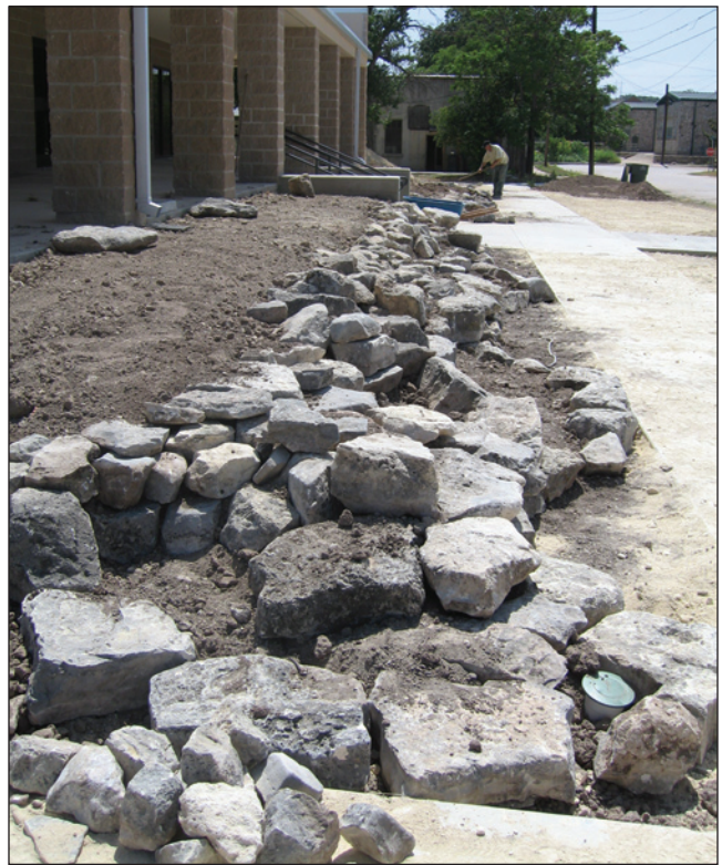
Final landscaping over a soil storage and infiltration system.
