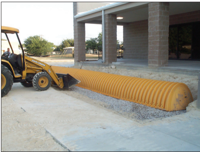
Installation of a soil storage and infiltration system.
