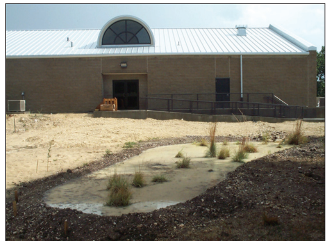
A recently constructed raingarden.
