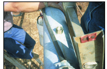
Figure 14. Swedge coupler installed.
