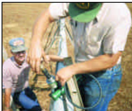
Figure 13. Installing swedge coupler.
