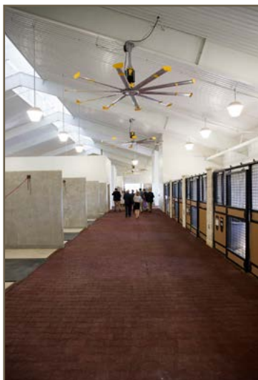
The aisles of the Equestrian Team barn feature non-slip rubber pavers, creating a horse-safe surface throughout the barn.
