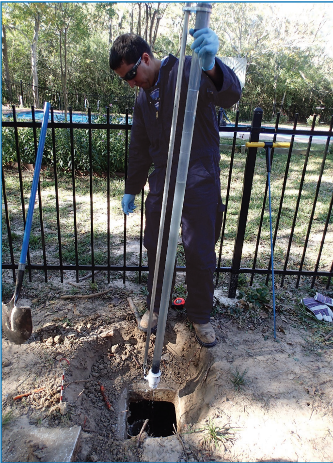
Figure 3. Inspecting scum and sludge layers inside the tank.
