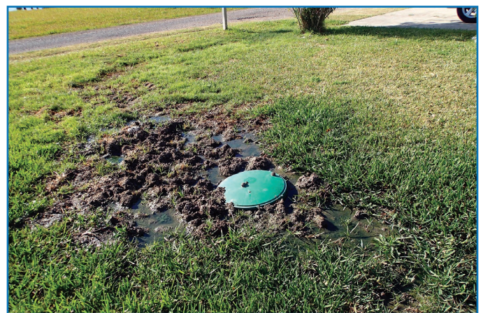
Figure 2. Surfacing effluent around a failing septic tank. Excessive vegetation, foul odors, stained soils, and saturated ground can indicate that the septic system is failing.
