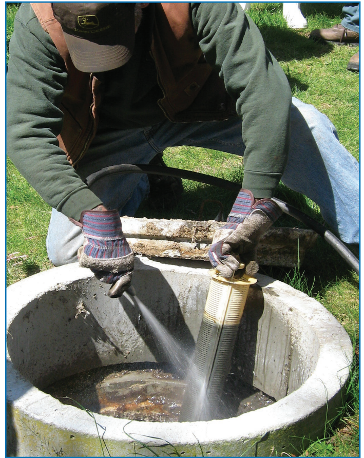
Figure 4. Cleaning an effluent screen over the inlet side of the tank. The riser installed on this tank allows quick access for maintenance activities.
