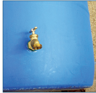
Figure 17. Hose bib facing down.
